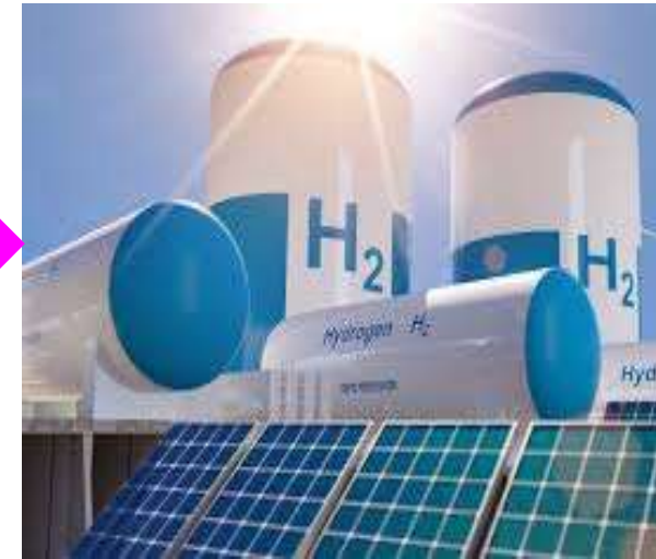
GREEN Hydrogen Production Plant Integrated into the 5MW FSPV
