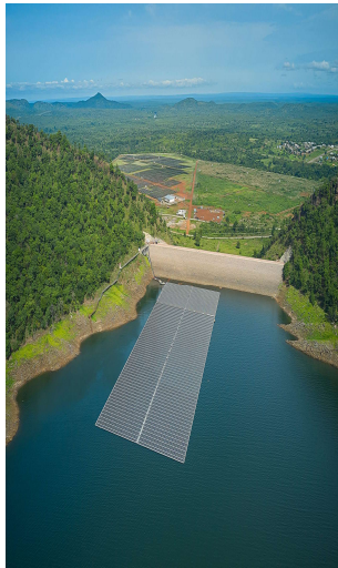
5MW Floating Solar PV Plant
