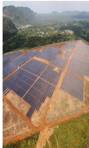
50MW Land Based Solar PV Plant
