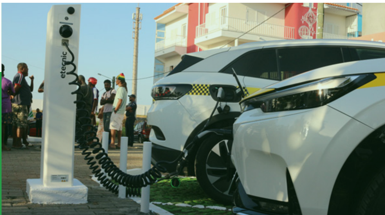
EV charging station in the Municipality of Santa Cruz in Cabo Verde Source: Ministry of Industry Commerce and Energy of Cabo Verde
