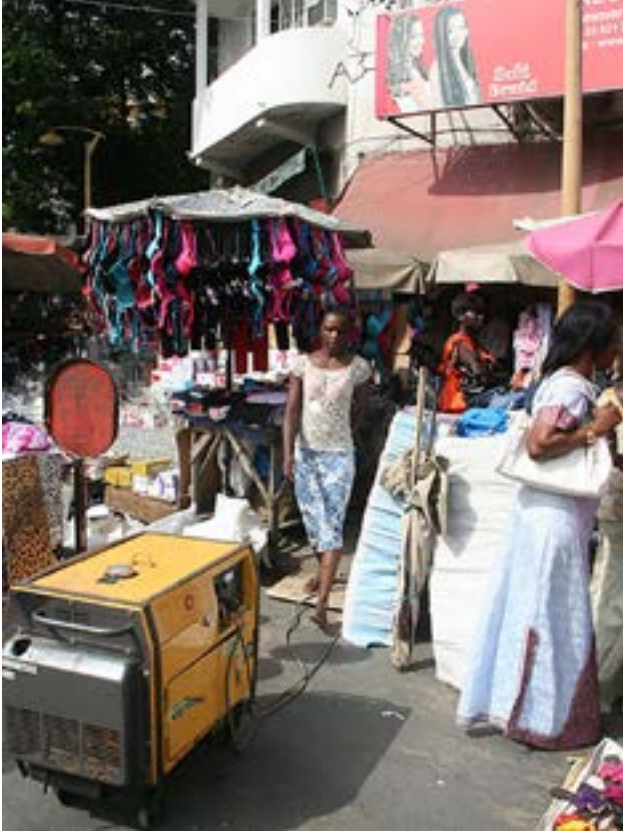
Generators are used by entrepreneurs to provide power during grid outages or to vendors without grid connections: Senegal
