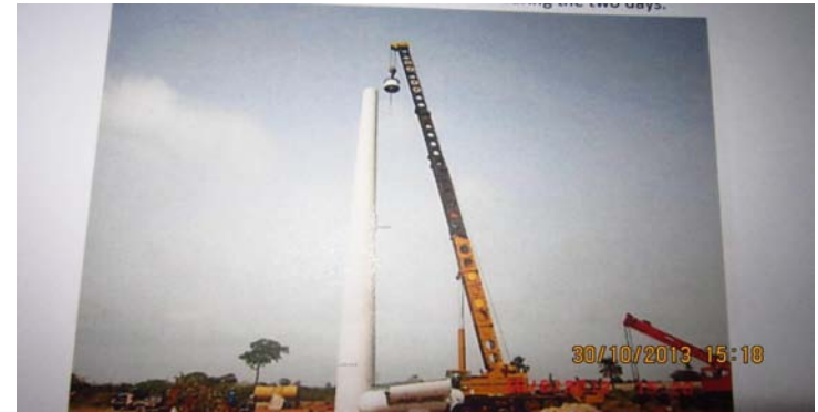
150 t crane at work turbin
