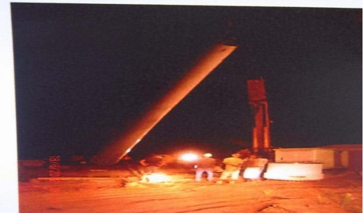
Works at night Wind Turbine
