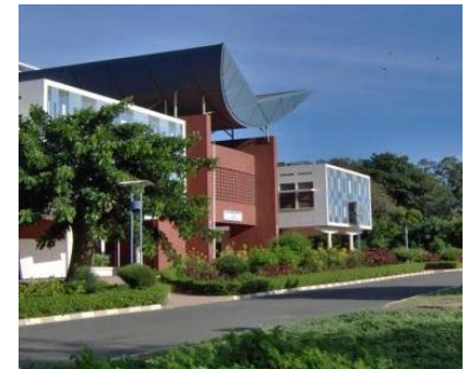
University building, Dakar (source: website of university)
