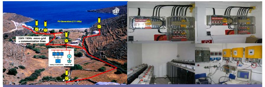
Load:12 houses connected on a single phase 230 Vac grid.Generation:5 PV units connected via standard grid-tied inverters.<br/>A 9 kVA diesel genset (for back-up).Storage:Battery (60 Volt, 52 kWh) through 3 bi-directional<br/>inverters operating in parallel.Monitoring:Data logging equipmentSource: NTUA, Greece
