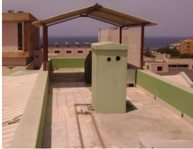
Analyzing the roof space
