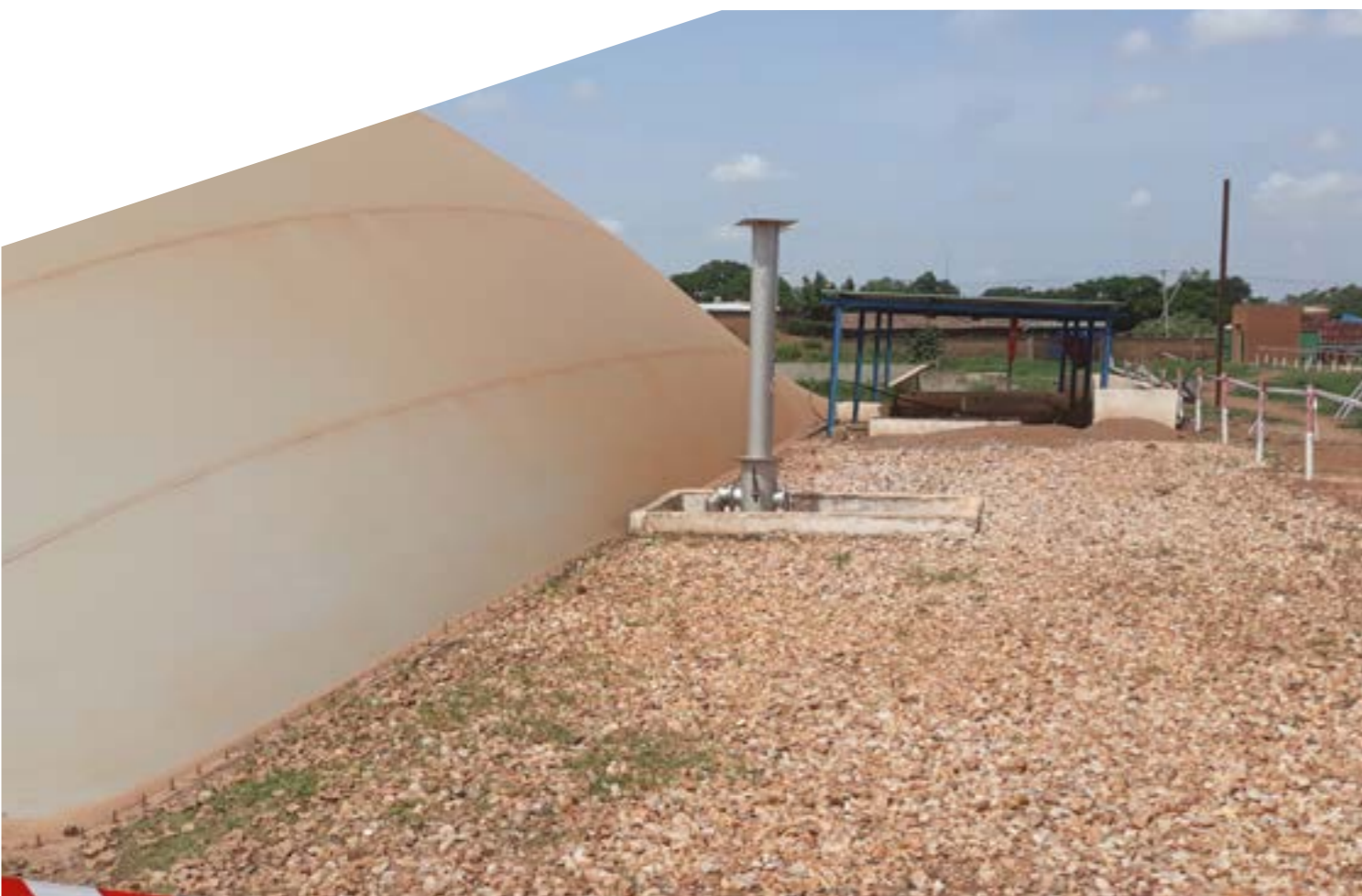
Lagoon digester with double-membrane
