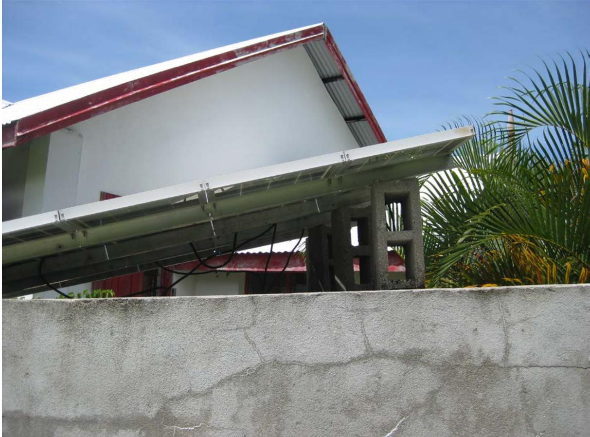
Answer: The array frame is not bolted down—it is being held up only by bricks.
