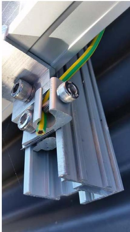
Answer: The insulation on the earth (ground cable) has not been stripped back to form a connection
